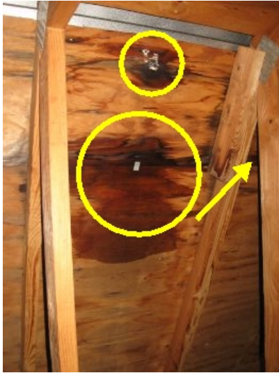
multiple roof leaks
