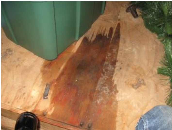
Leak from roof
